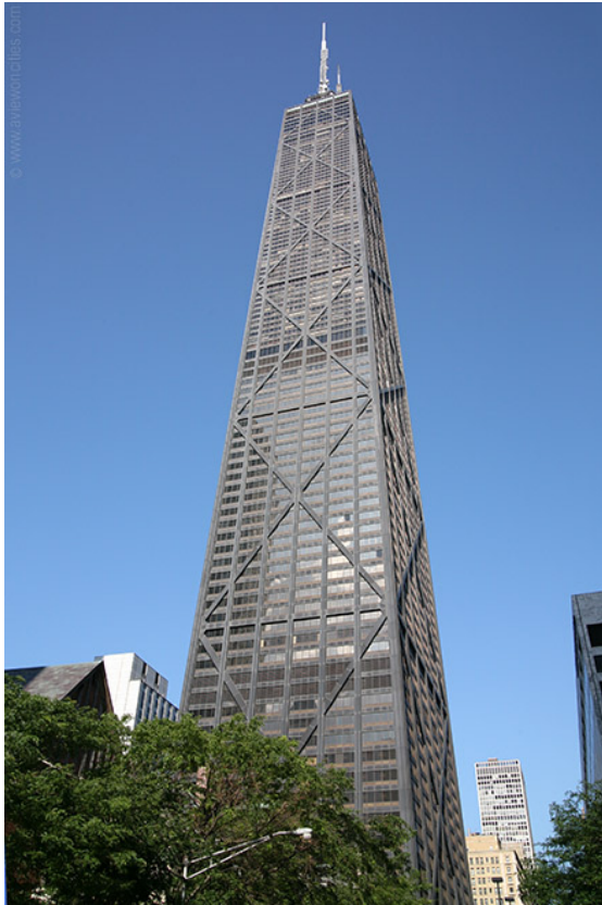
John Hancock Tower – Chicago 1969 (Skidmore, Owings & Merrill)
