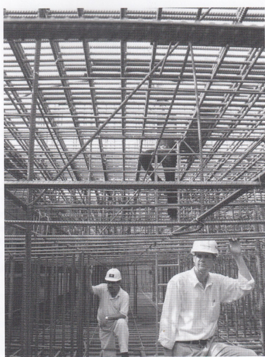
Mat Foundation Prior to Concrete Pour, Burj Khalifa, Dubai, UAE
