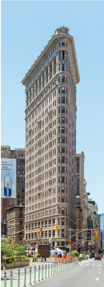
Fuller building (Flatiron) 1902 (Burnham - Dinkelberg)
