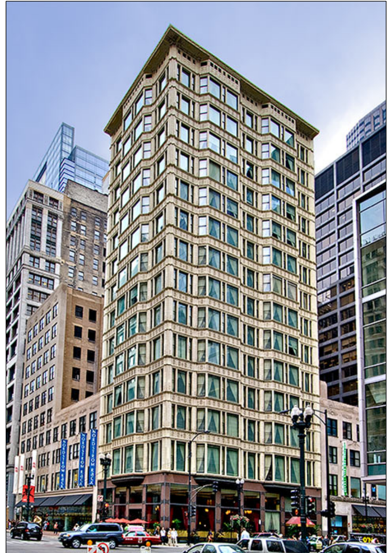
Reliance Building – Chicago 1891
