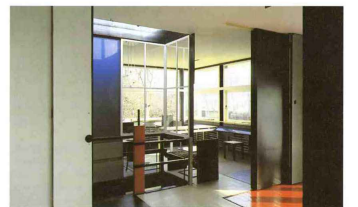
Above: plan of the first floor, showing sliding partitions closed. Drawing by Bertus Mulder, 1987 Below: same view as page 10, sliding partitions partly closed, and the movable window on the staircase railings in the position so that the living-dining area and stairwell/landing are separated from each other.
