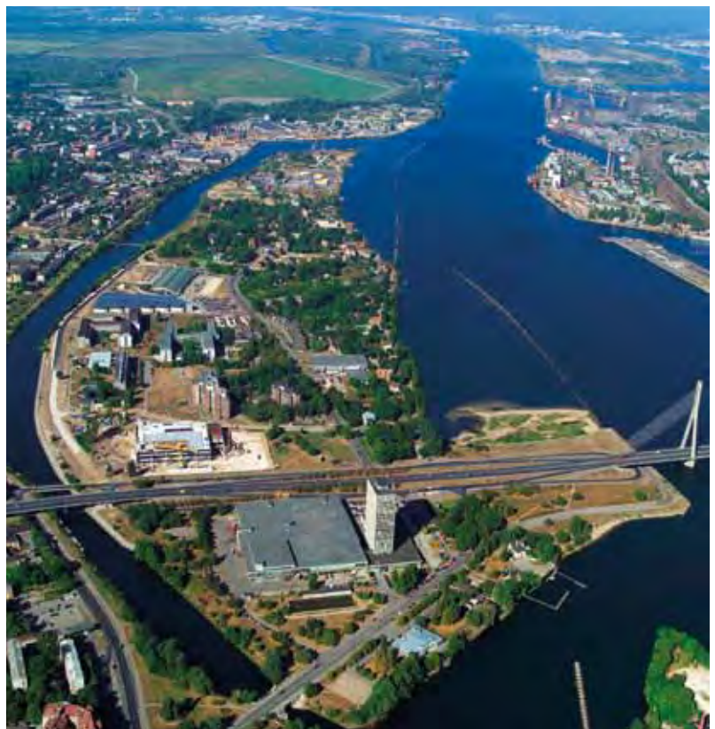
Aerial view of the River Daugava
