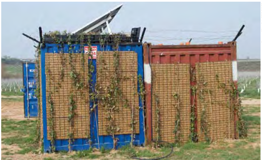
REAGRITECH built a hybrid wetland system using shipping containers and implementing hydraulic controls for recirculating water
